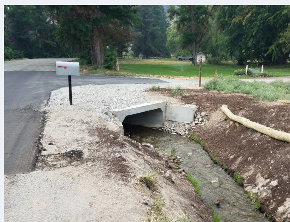
Culvert 3 before replacement. Photo Credit: Chelan County Public Works
