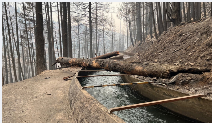
Trees and massive boulders crashed into the canal, damaging walls and weakening its structural integrity. Photo Credit (above and left): Yakima Tieton Irrigation District
