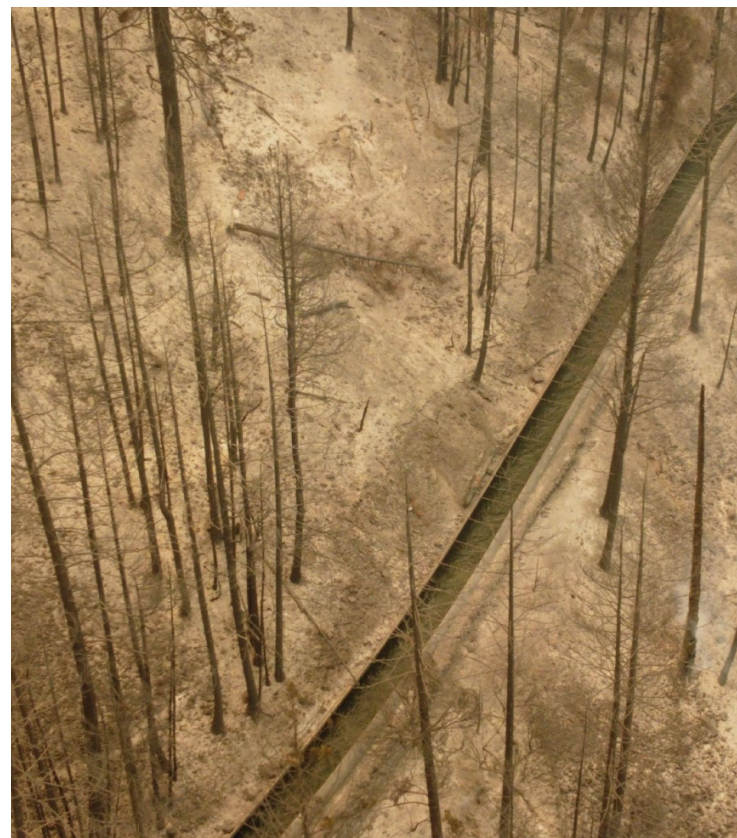
Trees and massive boulders crashed into the canal, damaging walls and weakening its structural integrity. Photo Credit (above and left): Yakima Tieton Irrigation District
