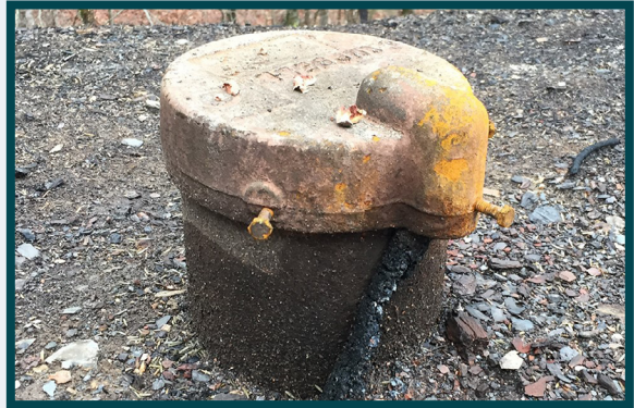
A fired damaged well cap. Photo: Center for Disease Control.
